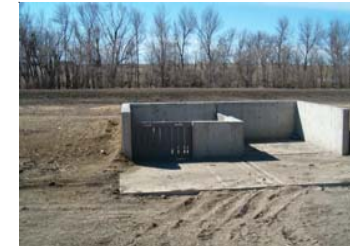
5) Runoff Evaporation Pond collects dirty water running off lots and is designed to evaporate a large portion of the incoming water.
