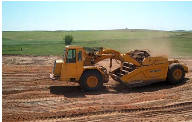
Construction phase of Ole Johnson's livestock waste containment system.
