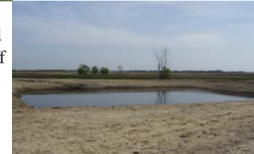
6) Solid Separator separates solids from lot run-off water and allows dirty water to run into the evaporation pond.
