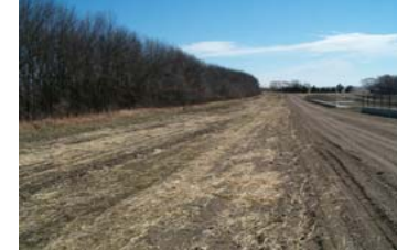
4) Clean Water Diversion reduces runoff and sometimes is the only management practice needed in small operations.
