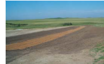
5) Runoff Evaporation Pond collects dirty water running off lots and is designed to evaporate a large portion of the incoming water.
